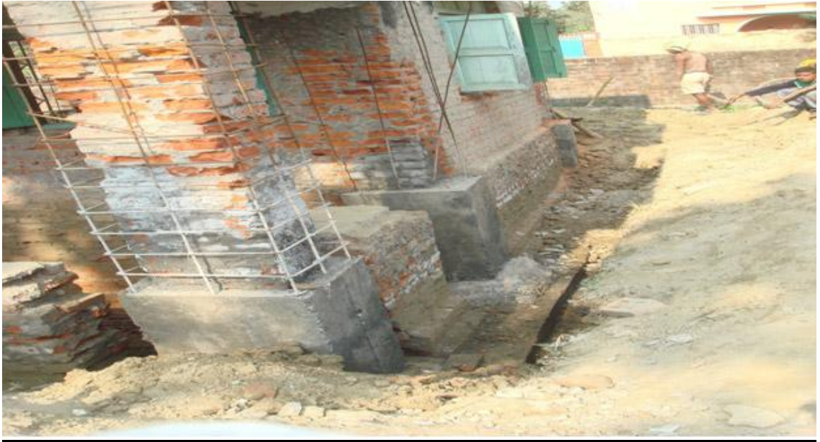
Laying of Reinforcement for Splints
