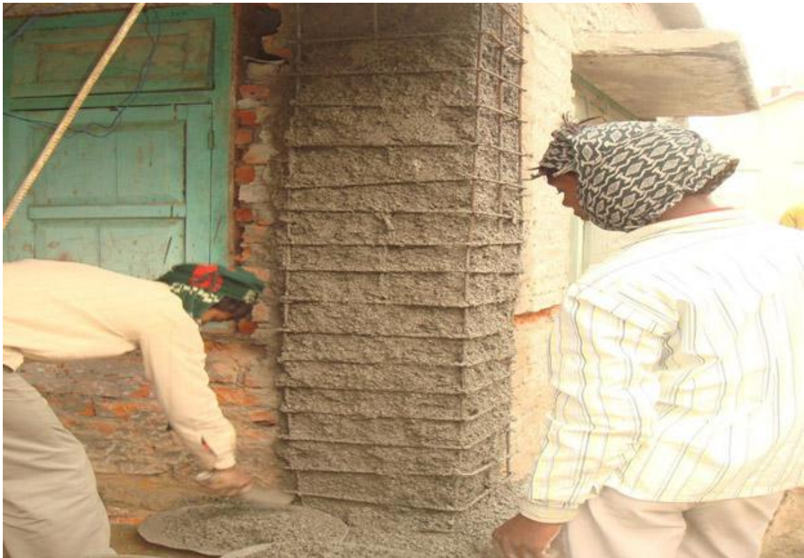
Micro- Concrete Work in Progress
