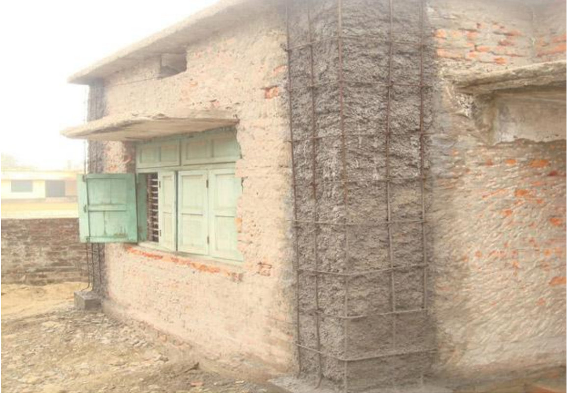
First Coat of Micro- Concrete
