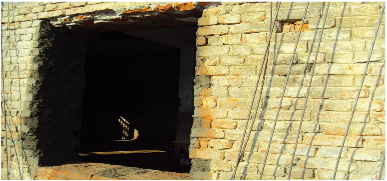
Window Removed for Replacement at South Face of the Building.
