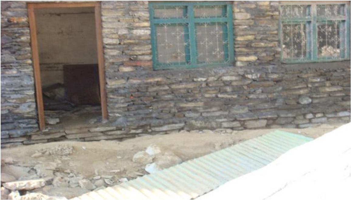
New Stone Masonry Work
