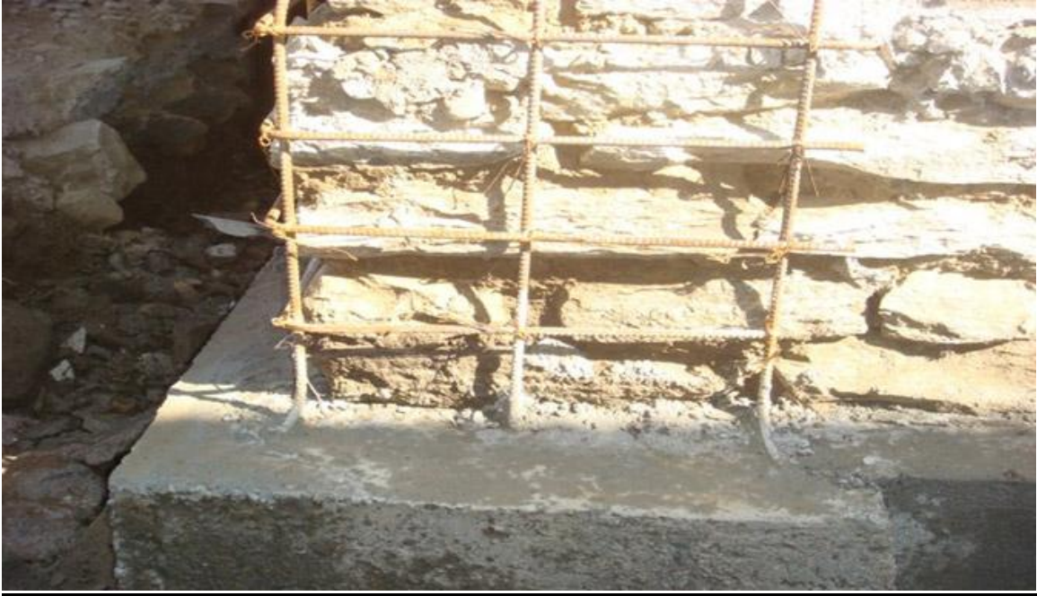
Reinforcement for Splint
