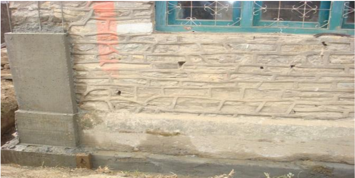
Micro Concrete for Splint
